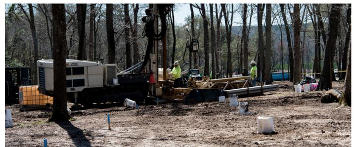
Department of the Air Force environmental restoration contractors use a geoprobe rotary sonic drill rig to drill a small diameter pipe into the ground at Sans Souci Farm in Sumter, South Carolina, March 7, 2019. The pipes are conduits for the precise injection of the BOS 100 product.
